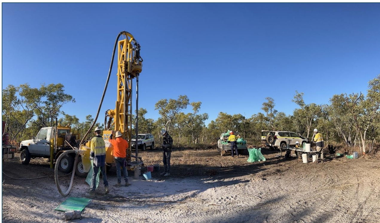
Figure 1: Drilling at Vanadis.
